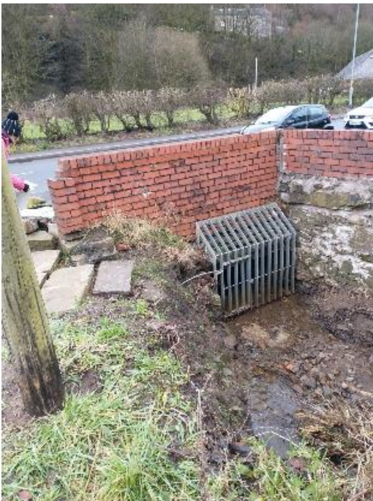
2025 culvert on the East side of the road looking toward the West
