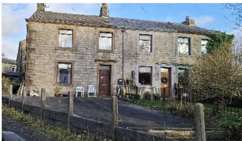
Above. SD 84242 25812 – (Top circle on map) House on Dean Road, formally an Inn called The Water Tavern. It has a datestone of 1831 but the owner confirmed that the datestone was added when the building was altered in that year and a third house was added on the right.
