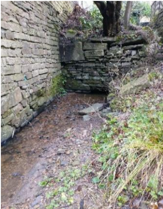
Culvert looking back towards the road
