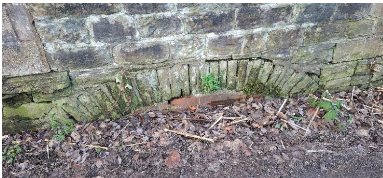
Above - Head race tunnel (sluice) and outside of northern wall
